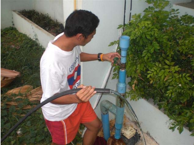
The water pump needs to be primed every time it is used and only needs a foot valve in the water tank.
